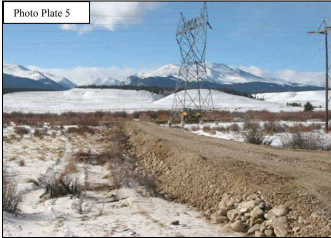
Photo Plate 5 Mt Massive Bypass during construction Note: High profile and cobble foundation
