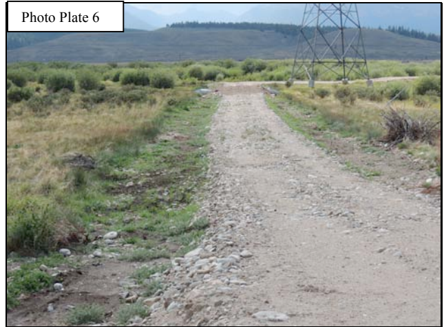
Photo Plate 6 Mt. Massive Bypass post-deconstruction Note: Reduced profile & width, exposed cobble at surface
