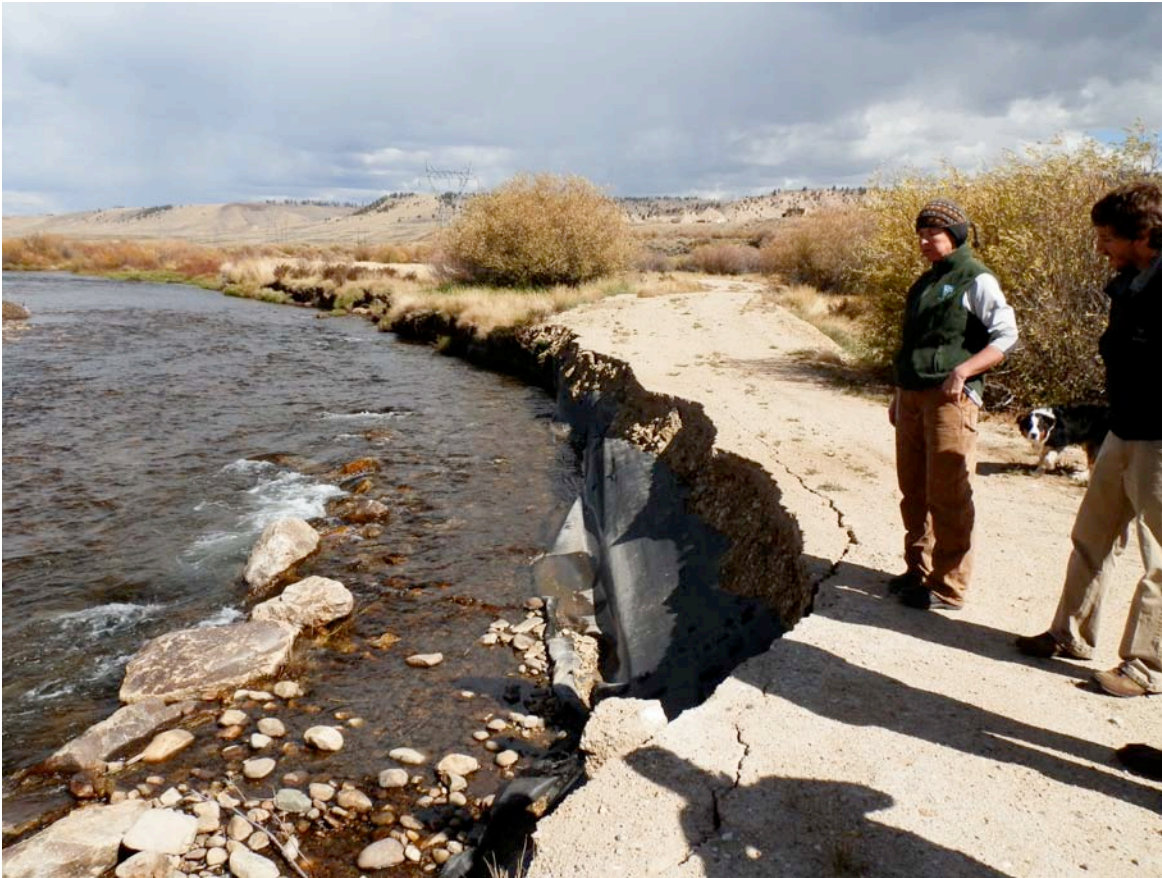
Photo Plate 13 Erosion of the EPA Haul Road caused by lateral migration of the river – October 2011 photo.
