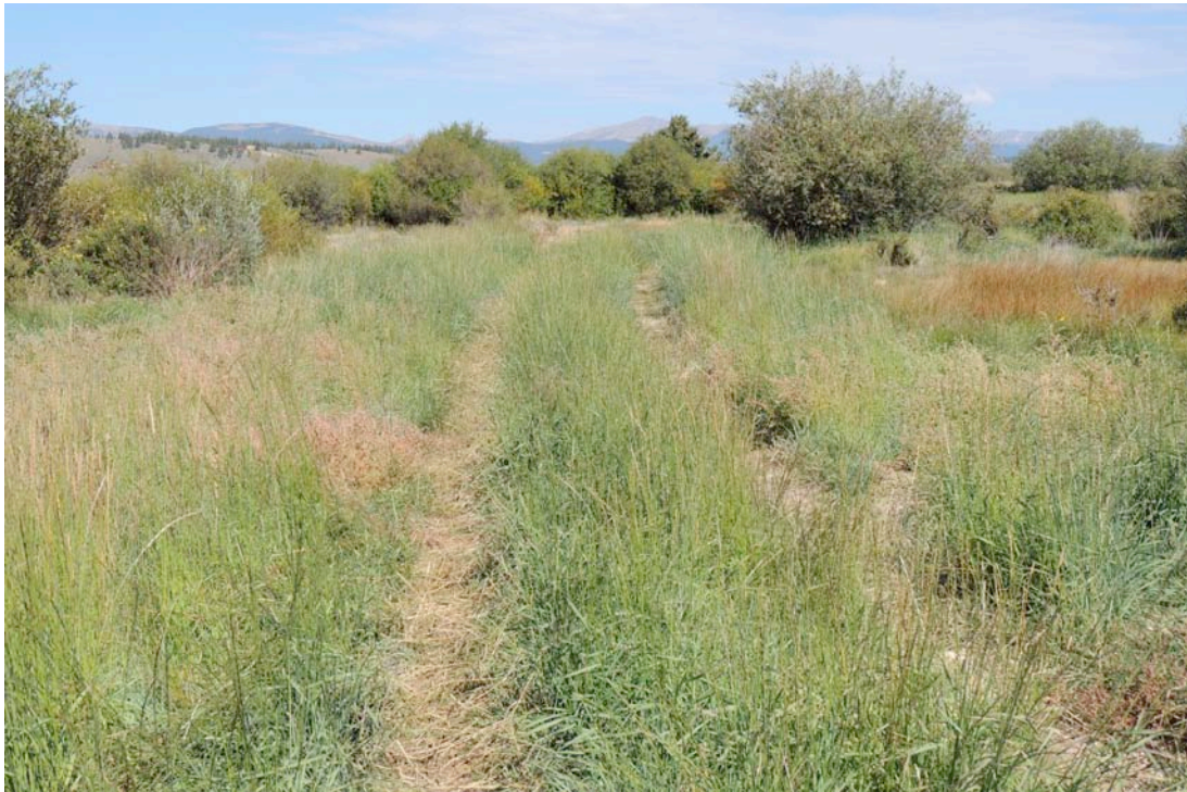
On-grade section of the reduced haul road where visual queuing and water control measures are not in place
